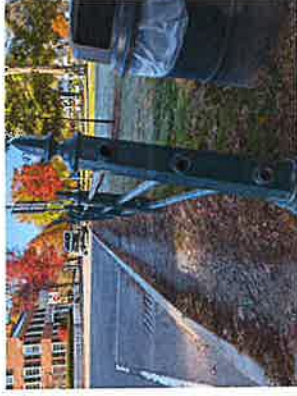
The fences are untrue and contain lead paint
